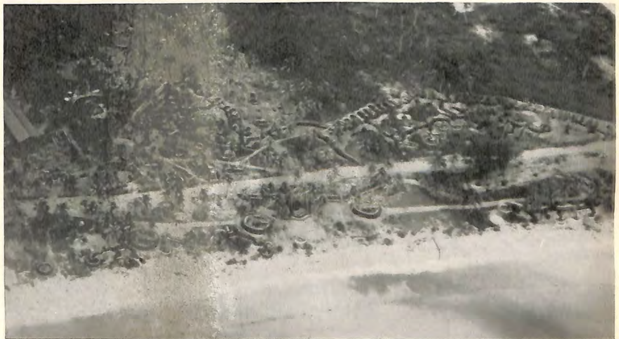
Figure 113. A typical coastal defense strongpoint.
